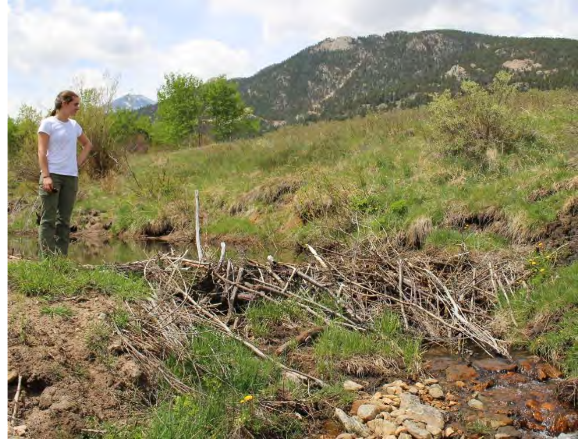
Beaver dam analogs (BDAs) Create mimicry structures to restore connectivity (e.g., Scamardo and Wohl, 2020)
